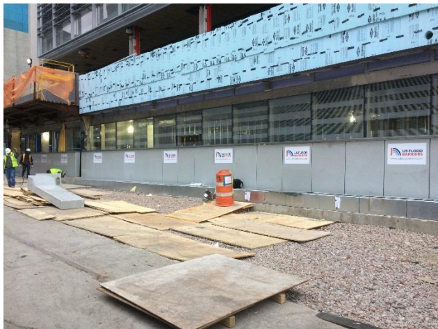
72m wide SAFB protecting Science Building main entrance.
