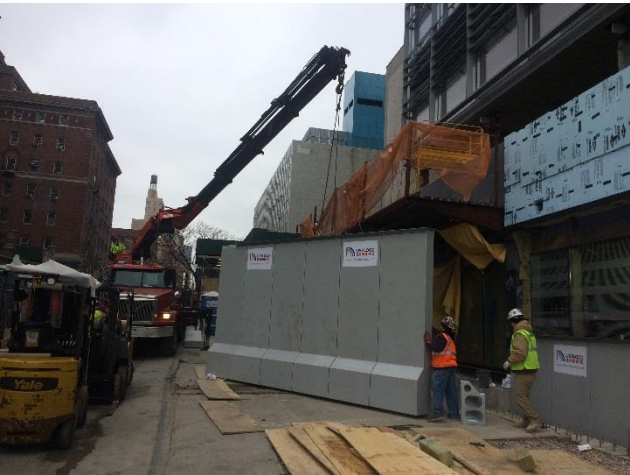
SAFB being installed. Barrier shown at 50% deployed.
